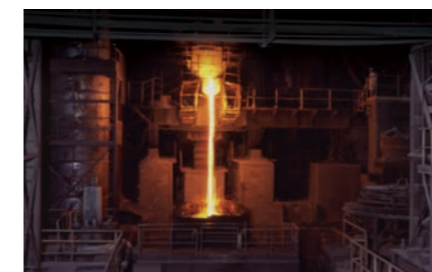
Electric arc furnace
